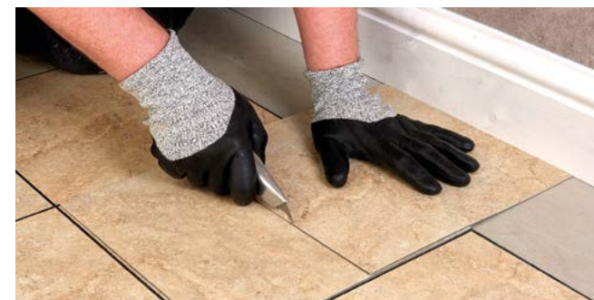
Figure 6 Measuring using an overlapping tile
