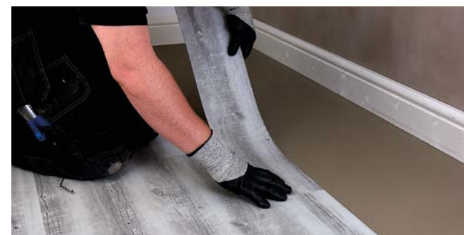
Figure 1 Setting planks out
